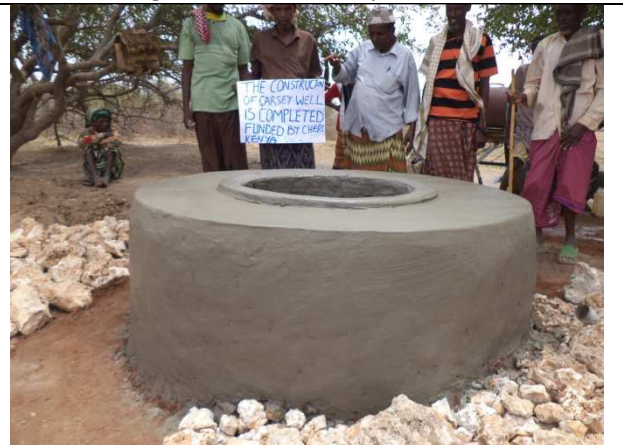
Well 'cupping' completed
