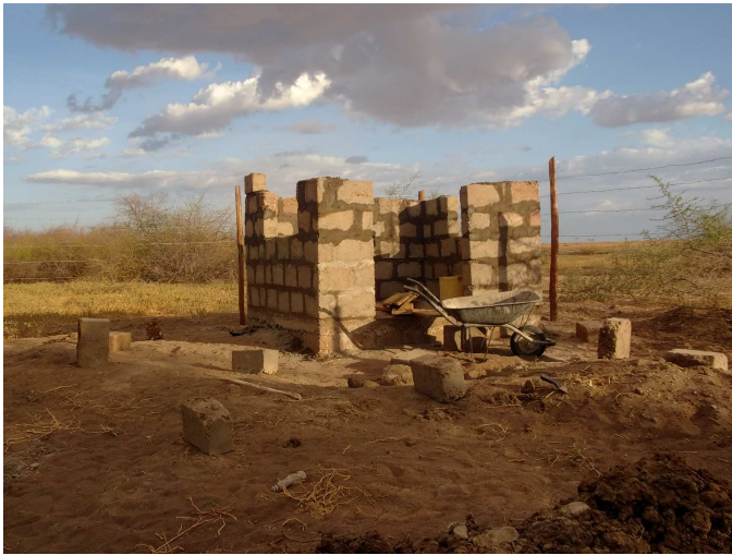
construction of pump house
