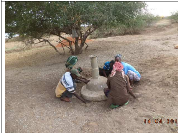
Old well top being removed
