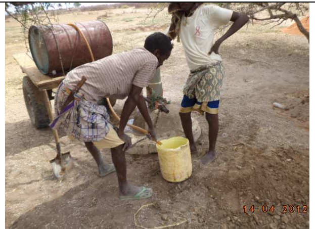
Water brought in barrel to help with construction
