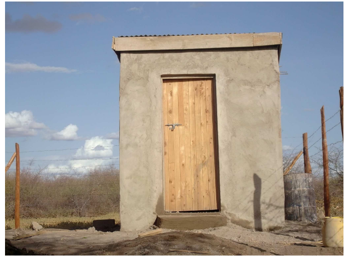
completed pump house ready for plumbing
