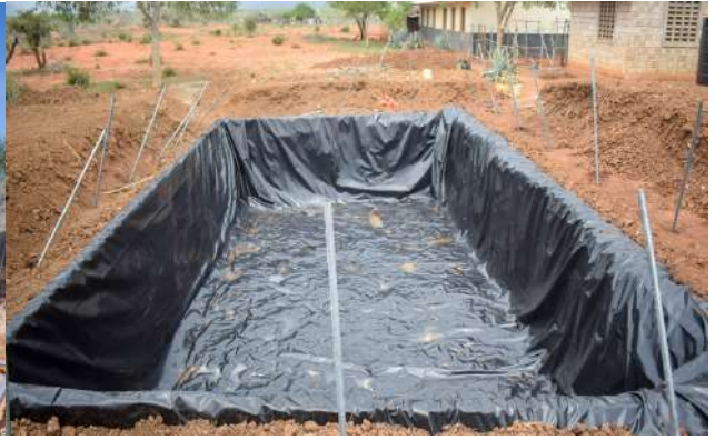
Sample of the 144,000 Litres water pans constructed in 3 villages of Chakama
