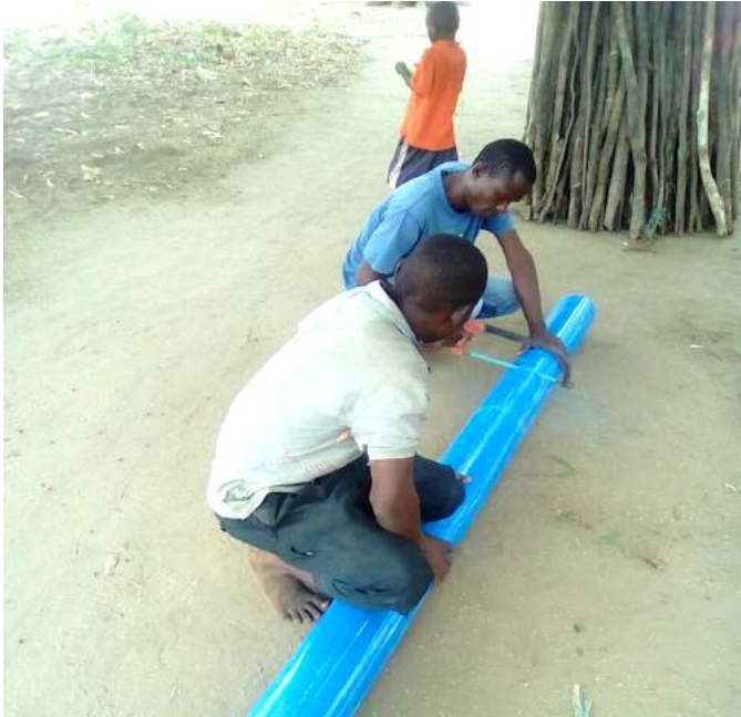
Cutting and fitting of casing pipes
